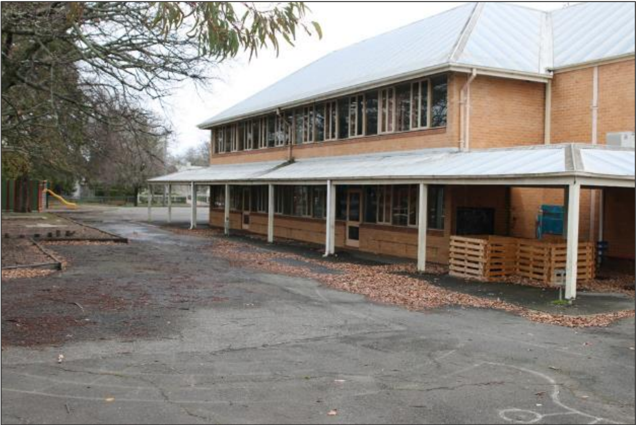
2G. Inside newer building extension
