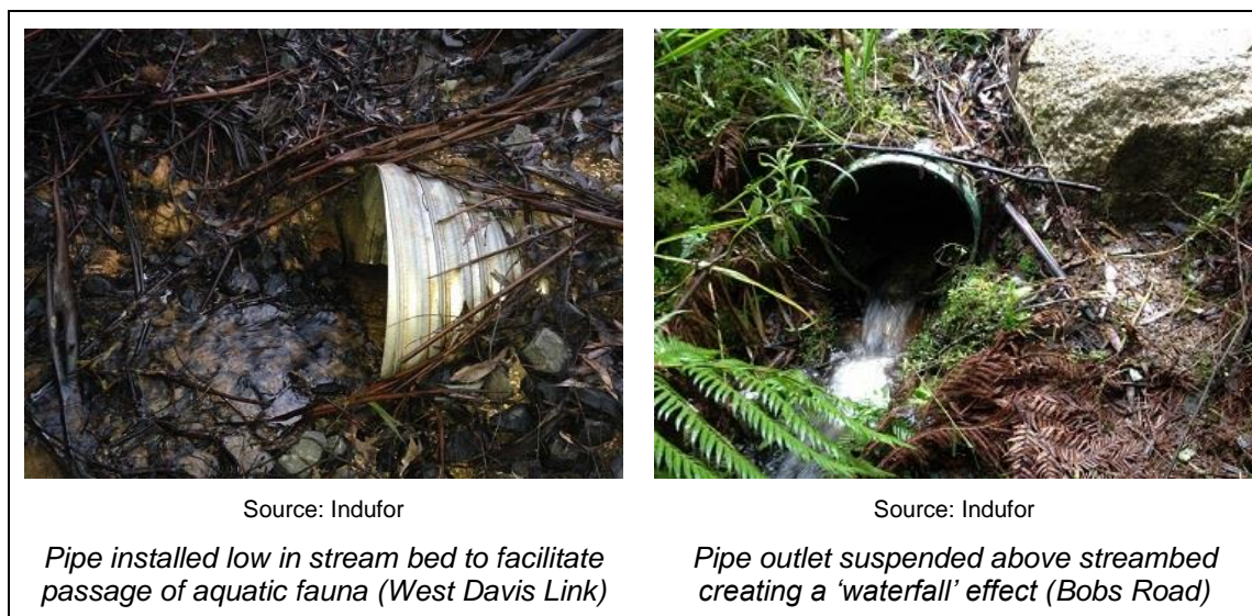
Figure 4-3: Pipe outlet positioning at the West Davis Link and Bobs Road coupes
