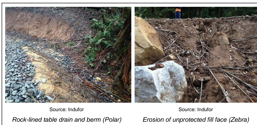
Figure 4-2: Rock-lined table drain and berm; and erosion of an unprotected fill face
