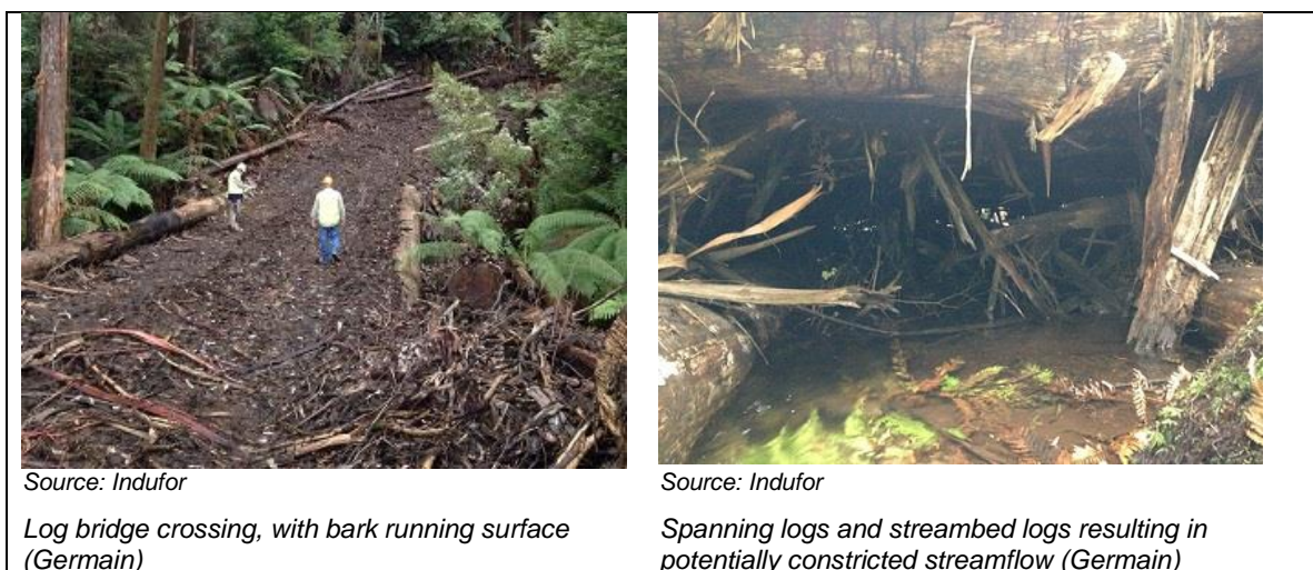
Figure 4-8: Germain snig track log bridge
