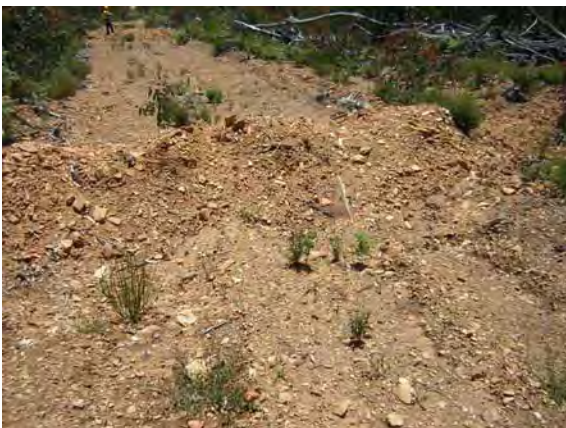
Photograph 17: Example of a well formed and effective snig track cross drain with outlet (C14).
