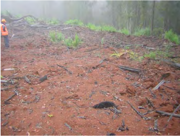
Photograph 15: Large area of rehabilitated landing without topsoil, associated with observations of poor topsoil segregation (C10).
