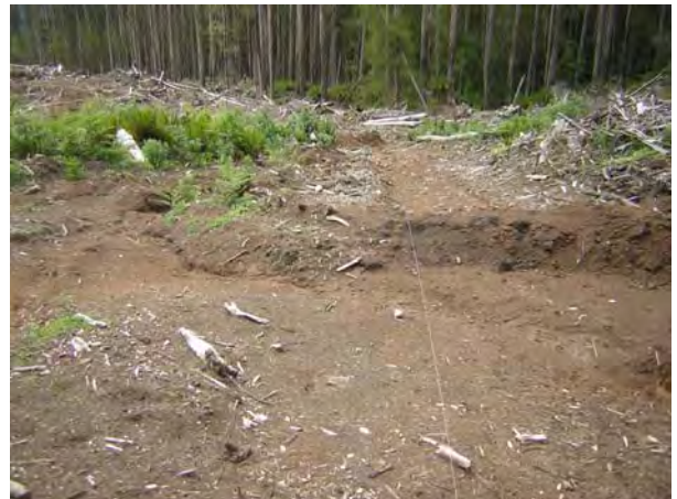
Photograph 19: Water flow around a bar due to no outlet channel on snig track drainage (C24).
