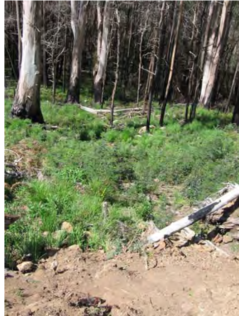
Photograph 9: Sedimentation below slumped cut slope (C20).
