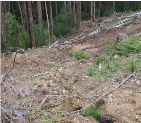
Photograph 8: Erosion in fill slope below cross drain outlet close to gully (C24).
