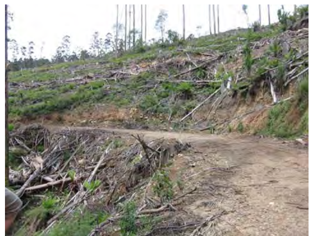
Photograph 6: Tree stump within minimum clearance width preventing full topsoil stripping and fill compaction (C24).
