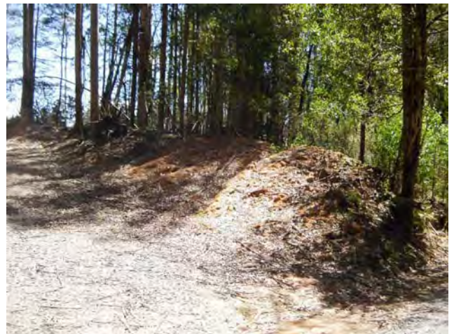
Photograph 10: Unplanned disposal of excess road construction fill within a rainforest buffer and pushed up around live trees (C3).
