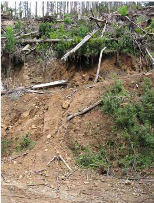
Photograph 12: Slumping and sedimentation in cut slope (C24).
