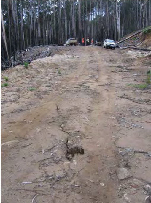
Photograph 11: Tension crack formed at cut fill line on in coupe road suggesting potential instability (C20).
