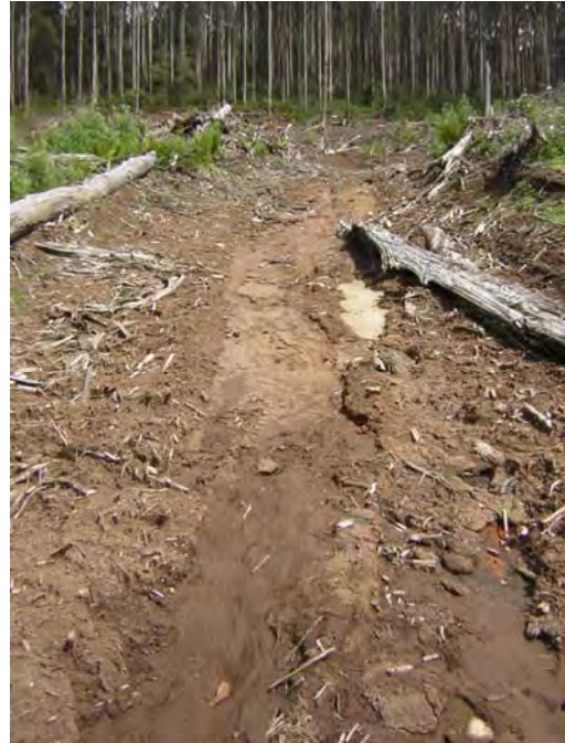
Photograph 18: Erosion of snig track due to inadequate drainage (C24).
