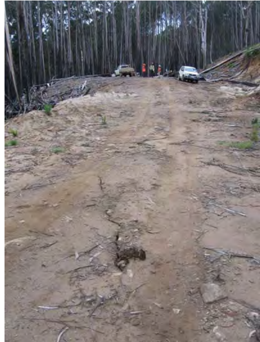
Photograph 13: Location of landing on ridge to minimise soil excavation. Landing also shared with an adjacent coupe (C20).
