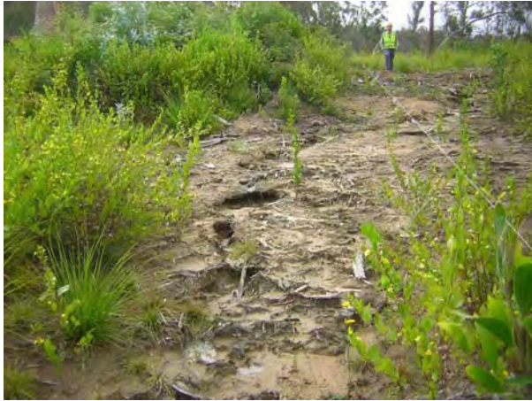
Photograph 20: Rilling of snig track due to inadequate drainage (C13).
