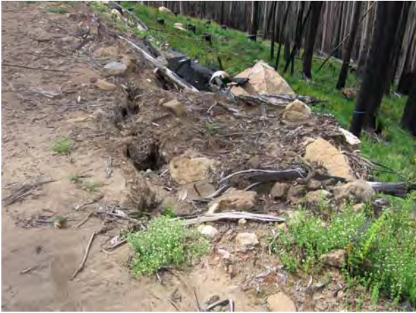
Photograph 7: Erosion of unconsolidated fill due to water flow (C20).
