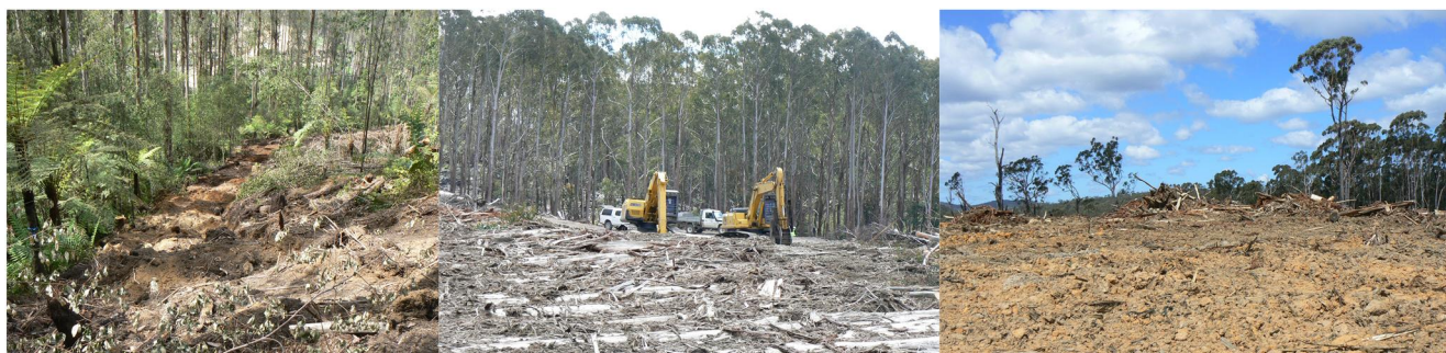
Coupe infrastructure: snig tracks are cross-drained progressively as harvesting proceed; active and rehabilitated log landings.
